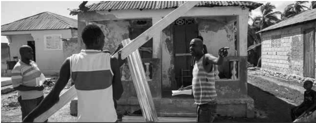
Hurricane Matthew devastated the southern half of Haiti. In some cities 80 percent of the houses were destroyed or damaged.
